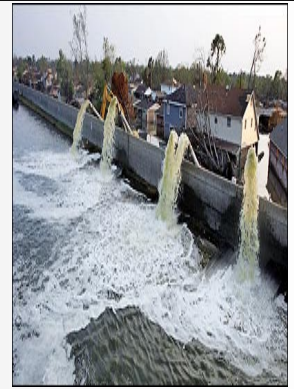
Pumps in New Orleans suck water out of flooded neighborhoods in September of last year after Hurricane Katrina swept through the city. The hurricane first hit the Gulf Coast on Aug. 29, 2005.
