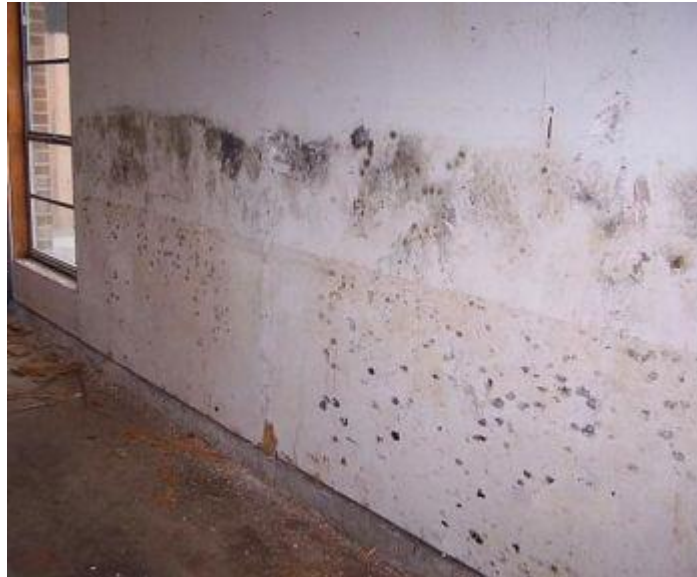
Black mold growing on the wall of a living room in a home that was flooded. (Marie Sanchez)
